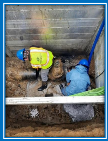
12 Inch Valve Replacement
