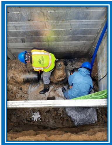
12 Inch Valve Replacement
